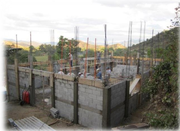
Construction of the Church building in 2014
